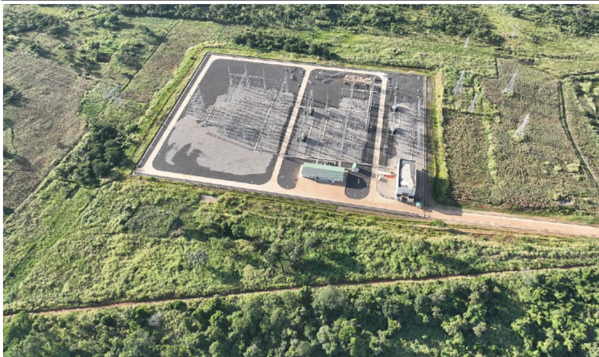
Figure 3-4 Existing Chipata West SS looking north-northwest
