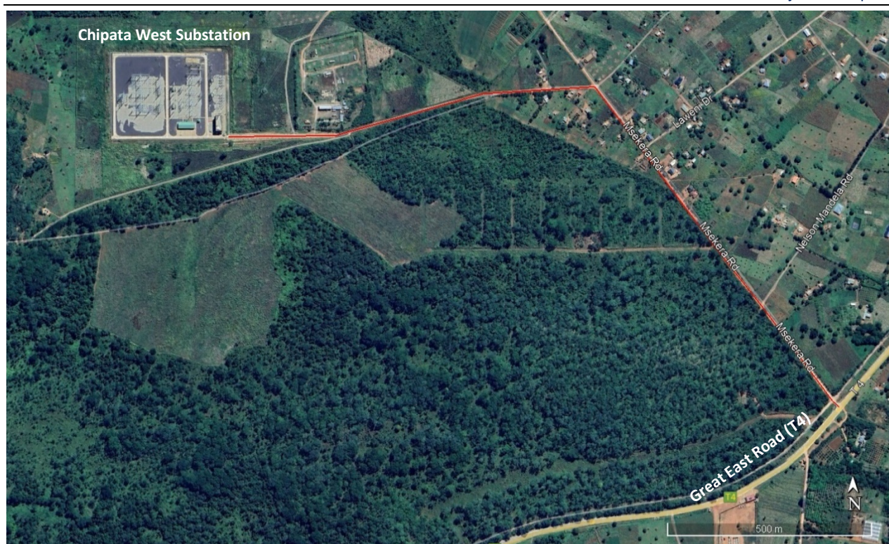
Figure 3-6 Existing access road of 1.9 km (red line) from the Great East Road (T4) to the Chipata West Substation
