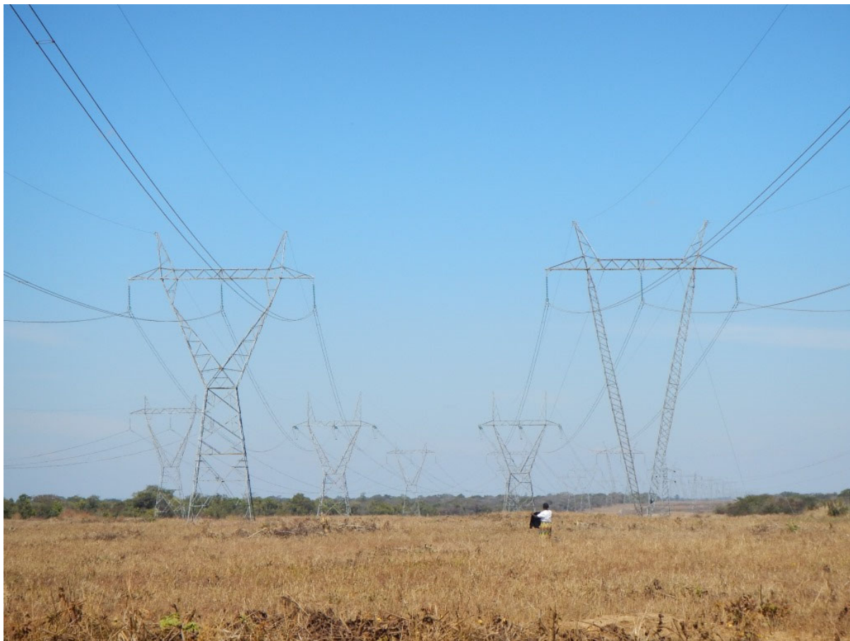
Figure 2-4 Combined Use of Self-Supporting and Guyed Single-Circuit Towers
