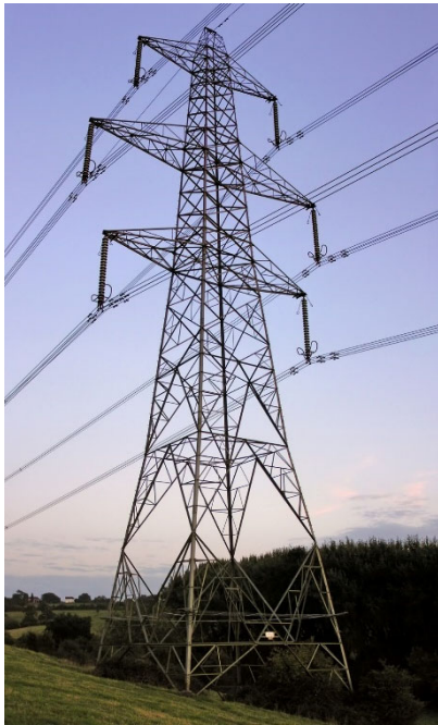
Figure 2-5 Typical DC suspension double-Circuit Towers
